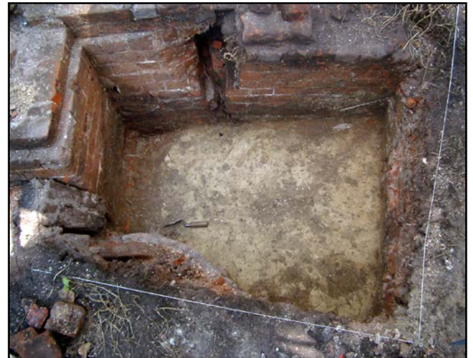
Figure 9: South wall (N505E300) and west wall (N510E295) showing cracks along the vent openings, and slumping of southwest corner of the structure.
