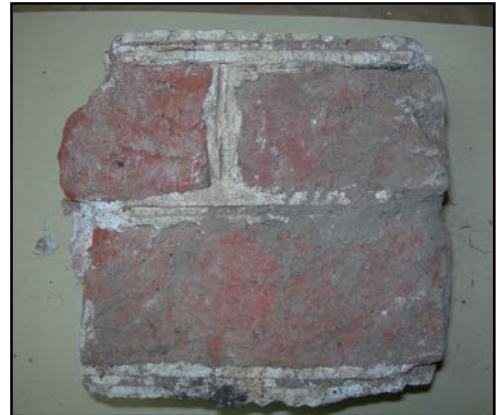
Figure 27: portions of intact brick showing struck mortar joint. Right is north profile of N510E290.
